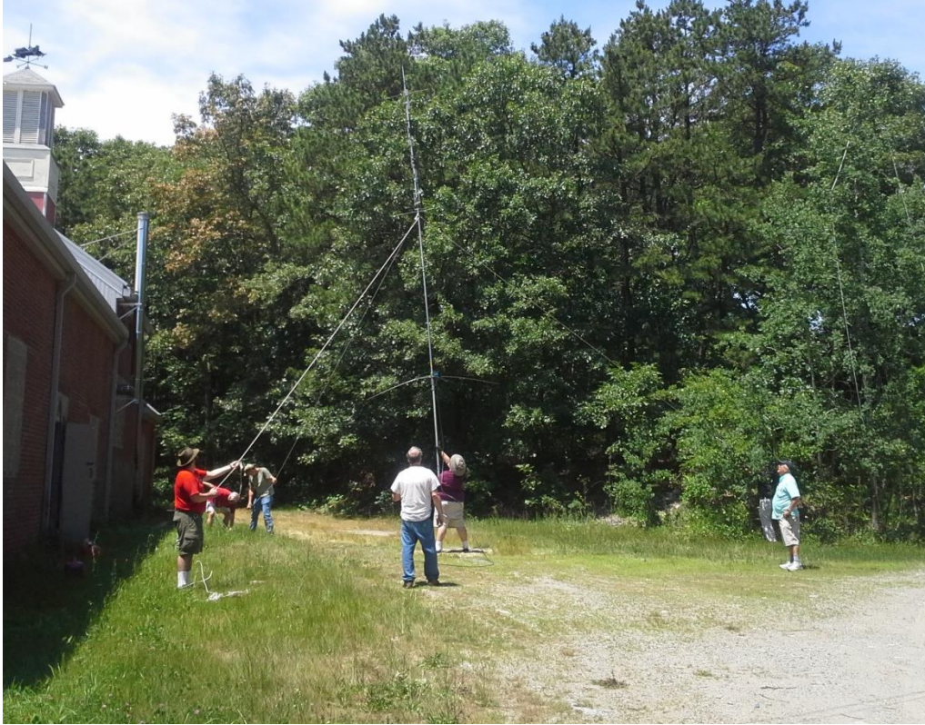
Raising the R7 vertical antenna
